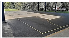
Resurfacing/line marking of the Secondary Multi-Purpose Shelter (MPS) with Synpave court surfacing
